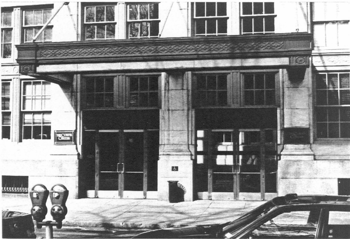
Figure 7. The Curtis Center, accessible entrance
