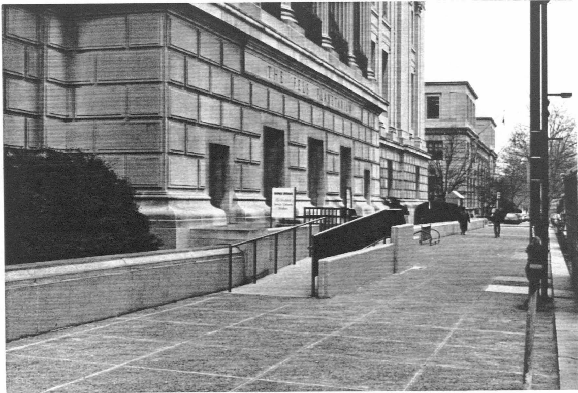
Figure 29. North (accessible) entrance to the Franklin Institute
