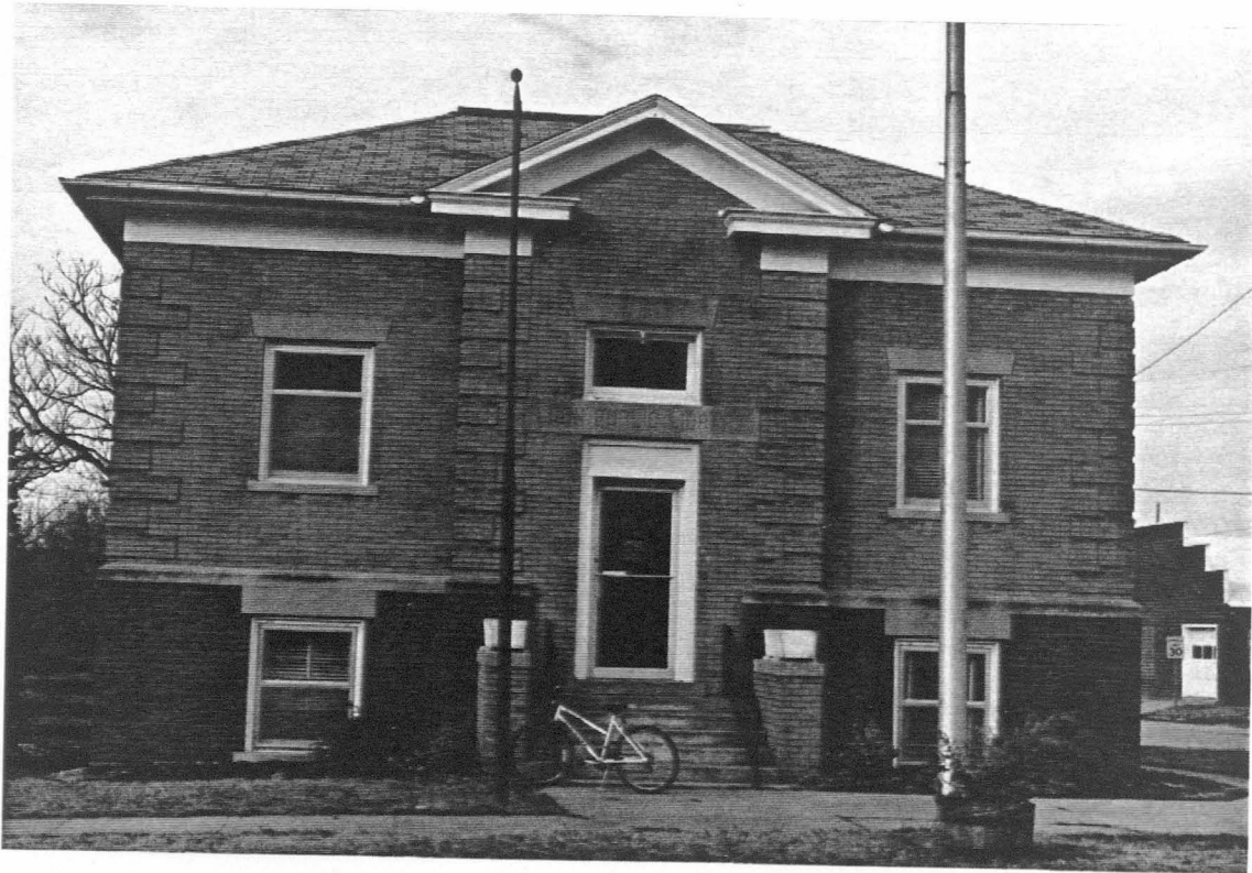
Figure 34. South view of Leon Public Library
