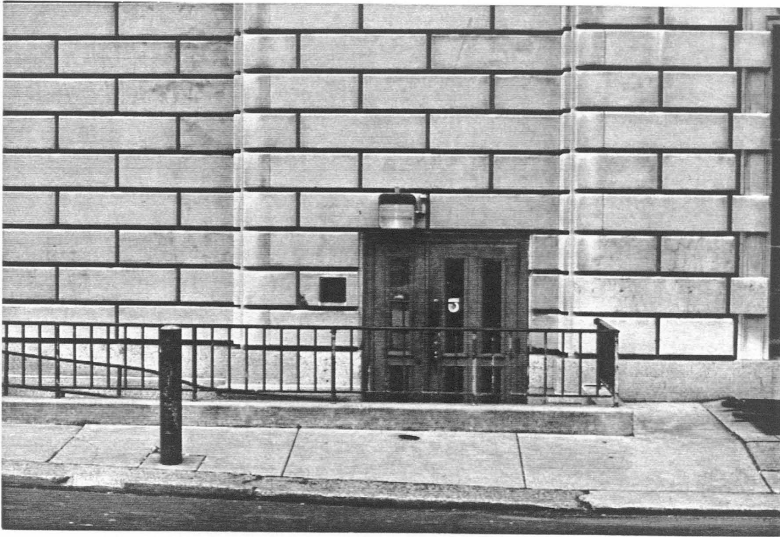
Figure 4. Free Library of Philadelphia, accessible entrance
