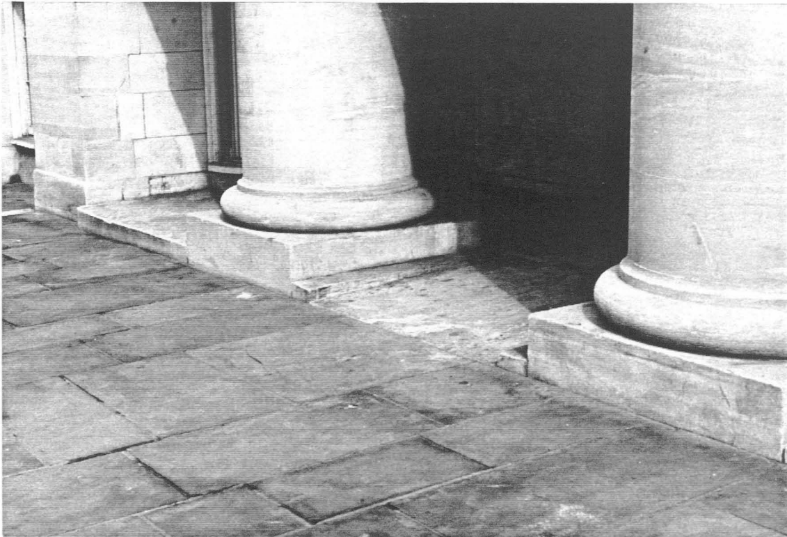
Figure 17. Detail of curb-cut in step at entrance of Merchant's Exchange
