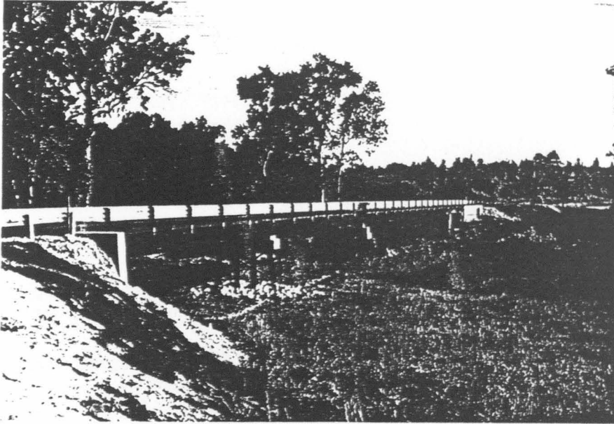
a) overall view of Wittson Bridge
