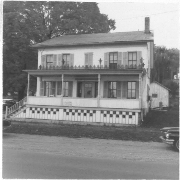
Figure 41. Smith House looking northwest
