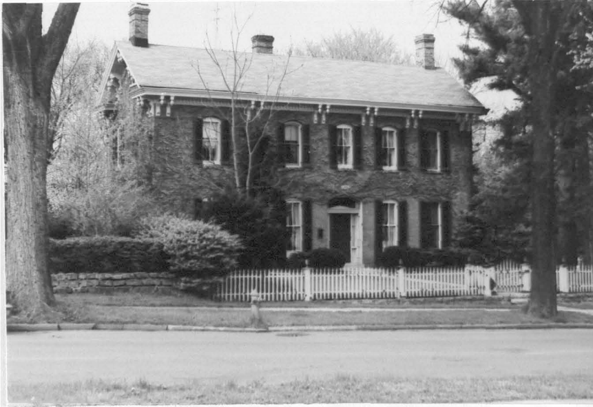
Figure 108. Grant Wood House looking north
