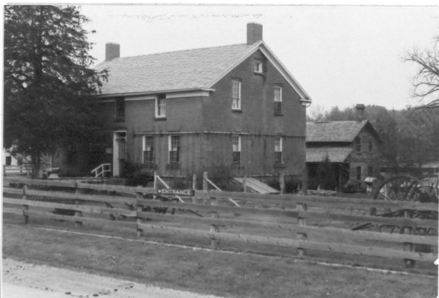
Figure 4. Amana Heim looking northwest with wash-house behind
