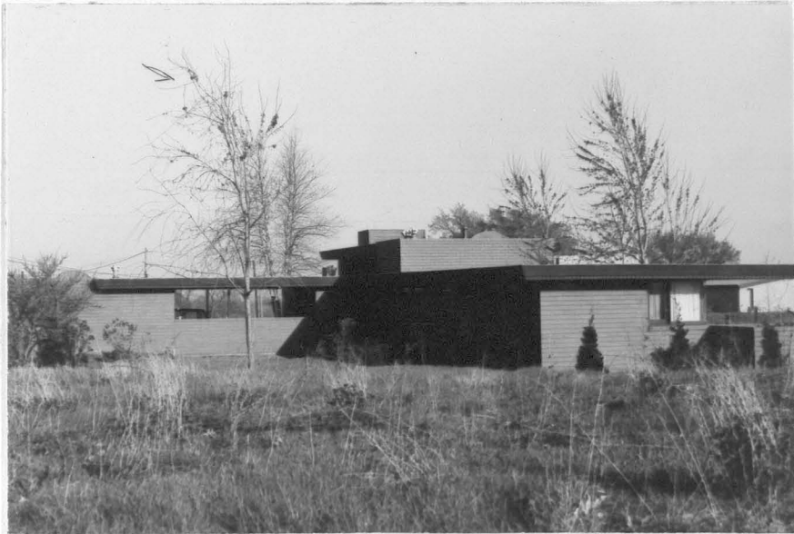
Figure 76. Trier House looking southeast with carport at left
