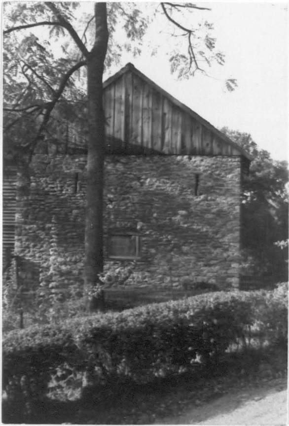
Figure 34. Miller House looking west at the barn
