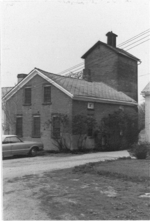
Figure 5. Smoke Tower looking northwest
