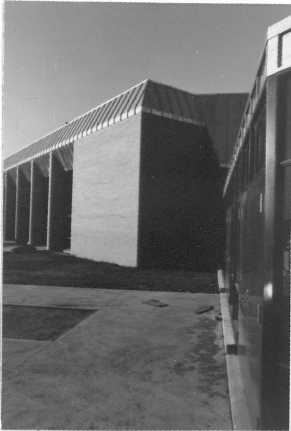
Figure 10. Gymnasium looking southwest
