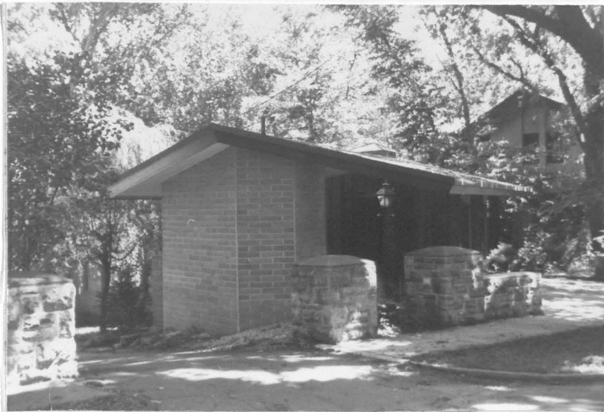
Figure 127. 15 South Rock Glenn looking southeast
