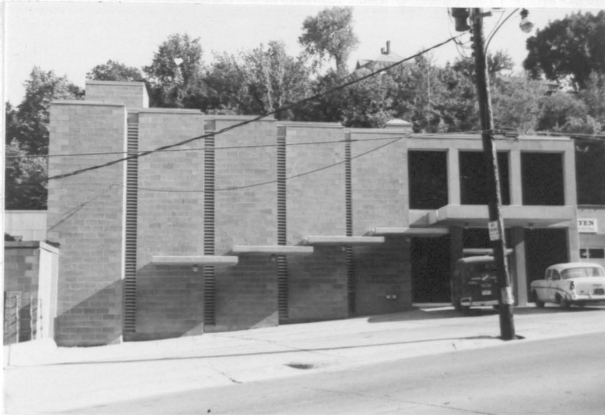
Figure 85. Lorenz Laundry looking south
