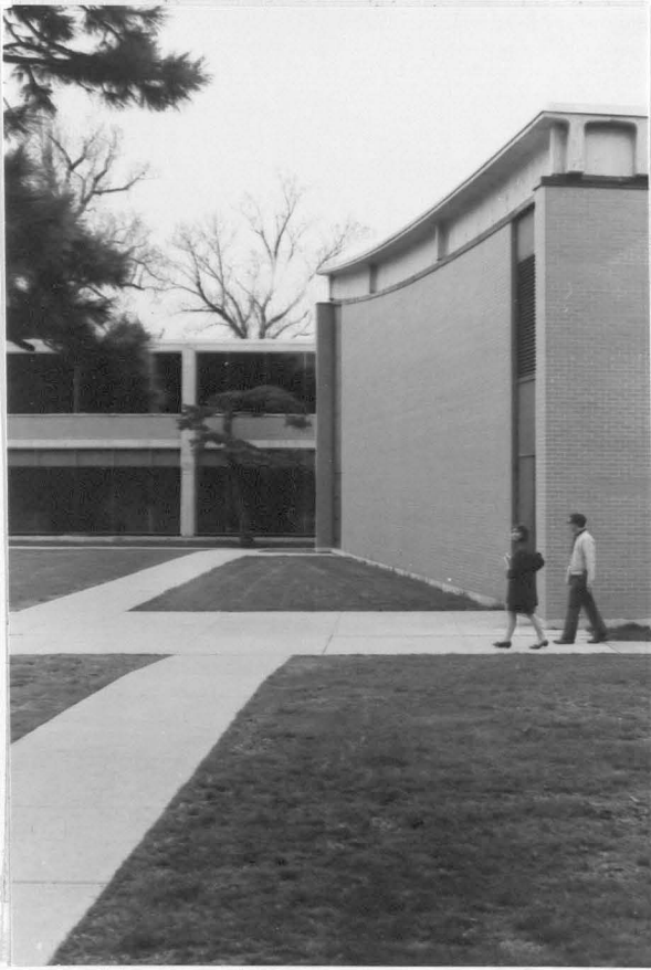
Figure 95. Roberts Theater looking south with Fine Arts at rear
