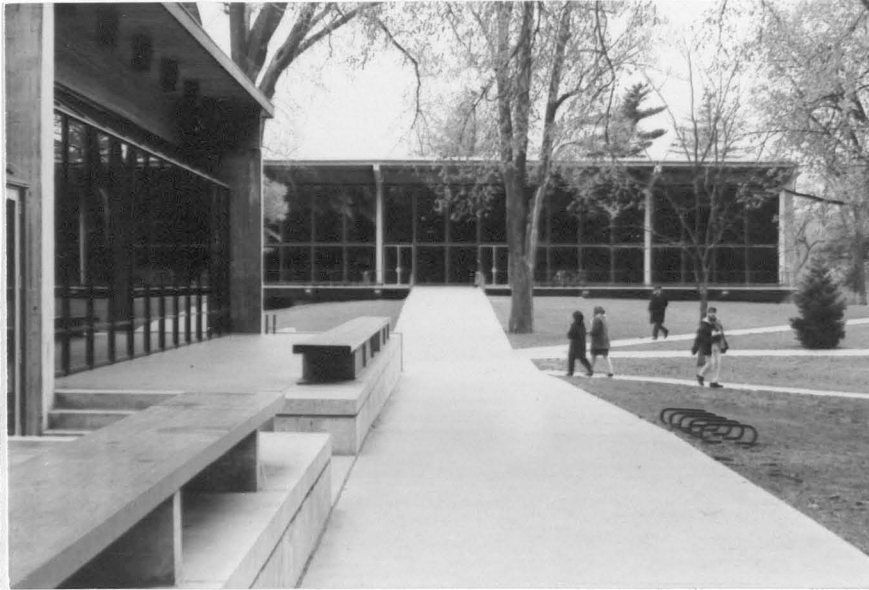
Figure 91. Burling Library looking south with Forum at left
