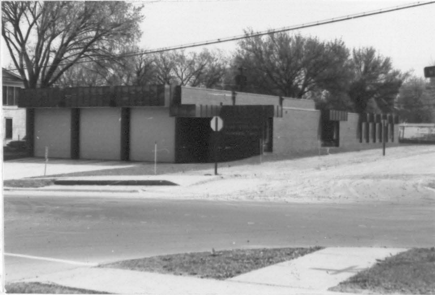
Figure 14. Fire Station looking northeast
