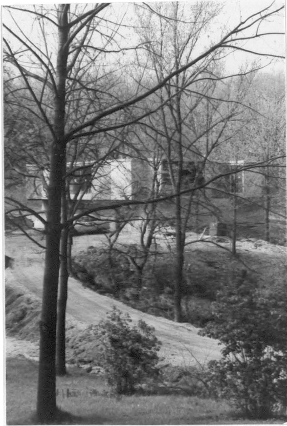
Figure 25. Hukill House looking north
