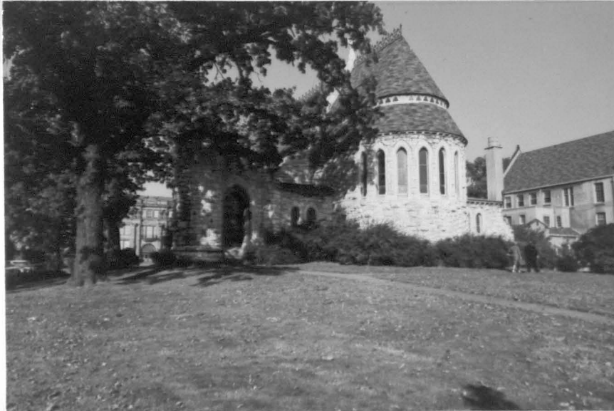
Figure 38. Trinity Episcopal looking west at the apse end
