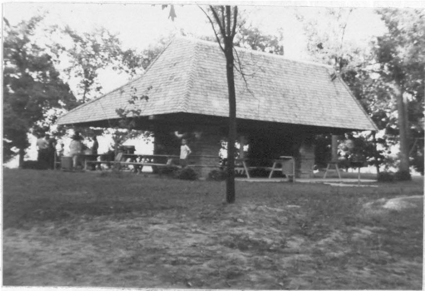
Figure 82. New Pavillion looking east
