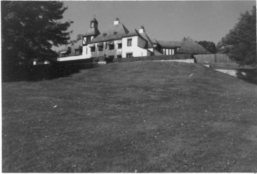
Figure 39. Capen House looking northeast at rear
