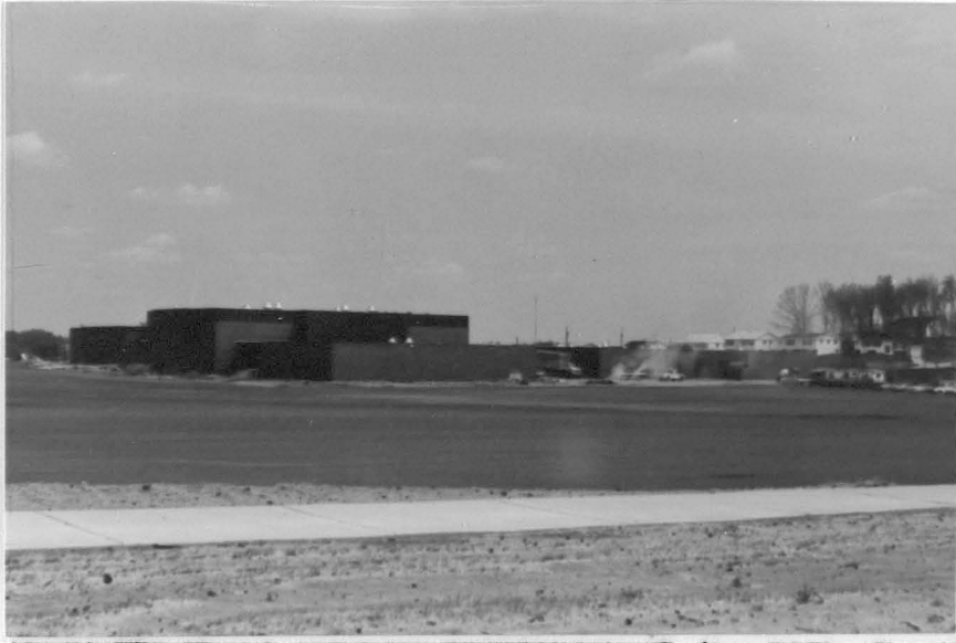
Figure 27. Kennedy High School looking north
