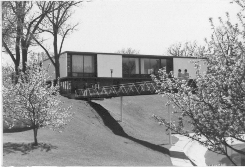
Figure 51. Dining Hall looking south
