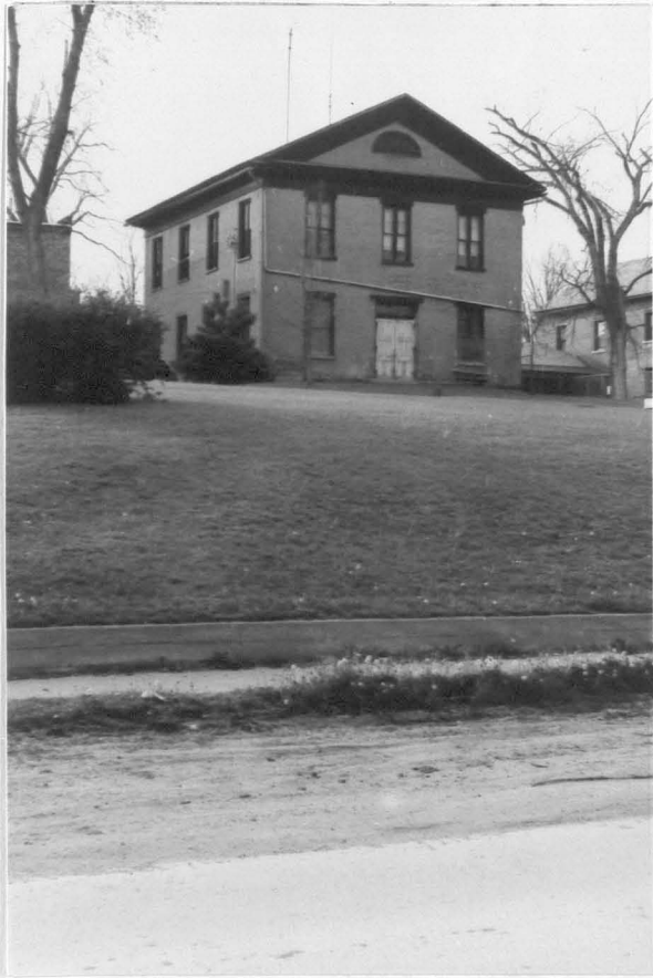
Figure 118. Van Buren County Court House looking north
