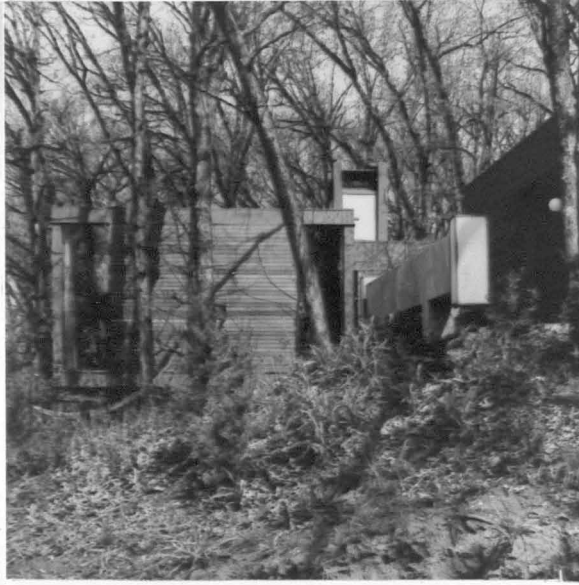
Figure 30. Shuttleworth House looking north
