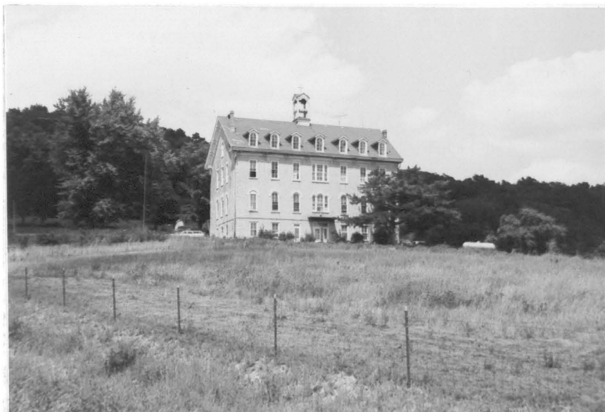
Figure 89. Residence looking north
