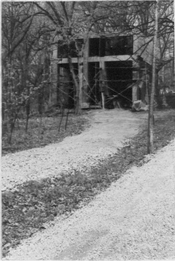
Figure 22. Farris House looking north
