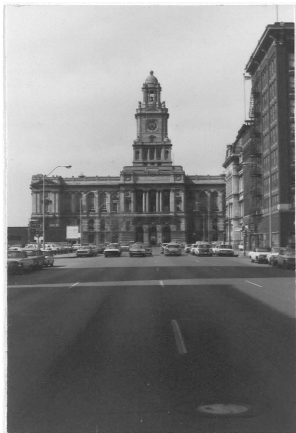
Figure 71. Polk County Courthouse looking west
