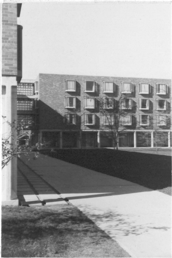
Figure 57. Men's Dormitories looking west into courtyard
