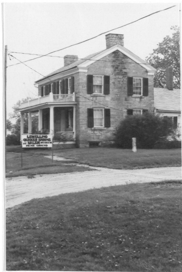
Figure 119. Lewelling House looking south
