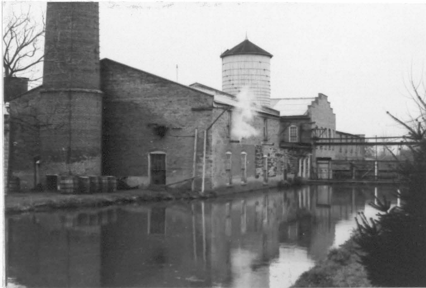
Figure 8. Hydro-electric Plant looking east across canal
