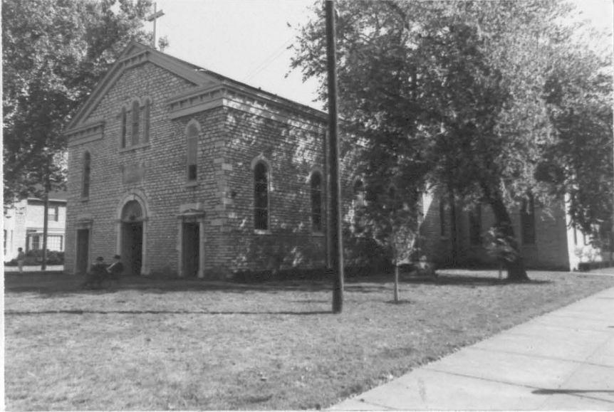
Figure 35. St. Anthony's Church looking northeast
