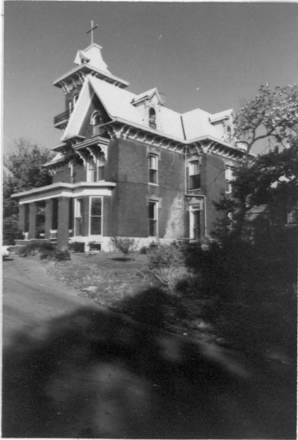
Figure 36. St. Katherine's Hall looking northwest
