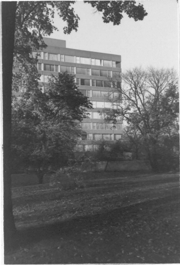
Figure 75. 3660 Grand looking northeast
