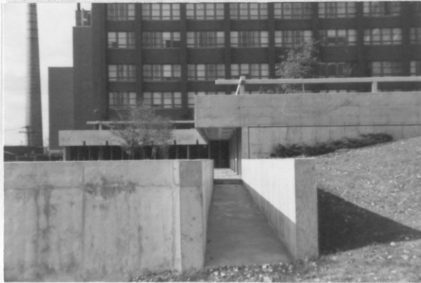
Figure 65. Looking west into first roof garden of Service Addition
