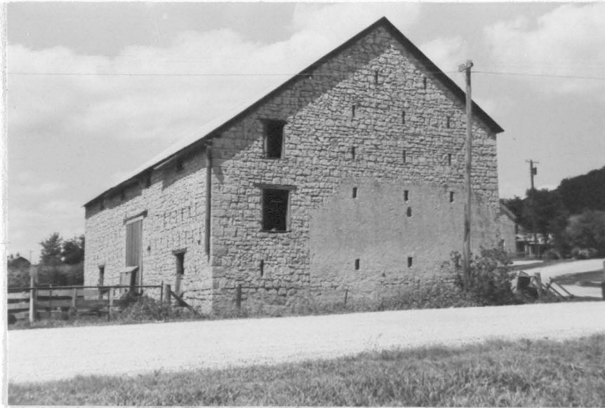
Figure 88. Barn looking north
