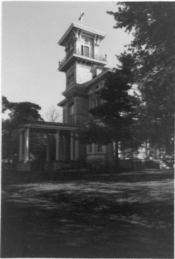
Figure 37. St. Margaret's Hall looking north
