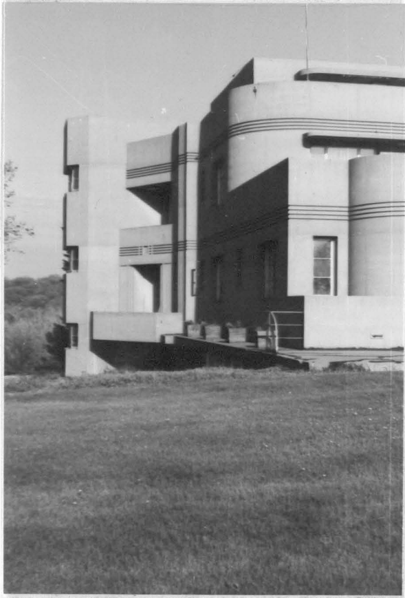
Figure 70. Open Bible College looking north
