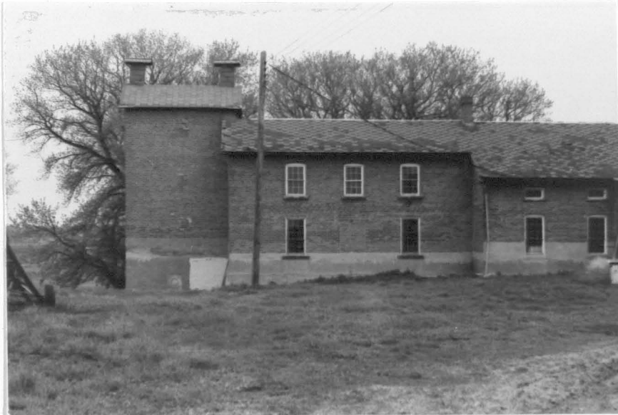
Figure 6. Factory looking east
