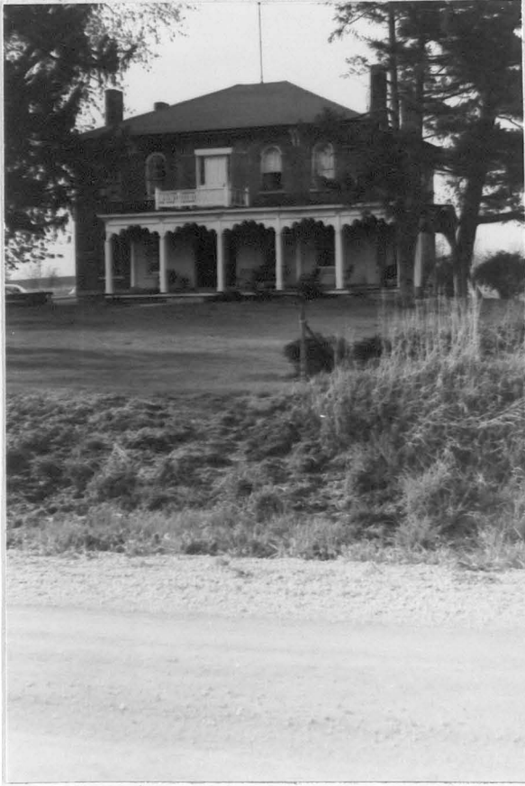
Figure 112. Meek House looking north
