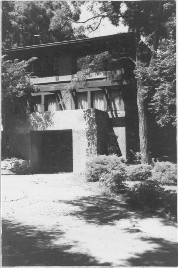
Figure 126. 11 South Rock Glenn looking south
