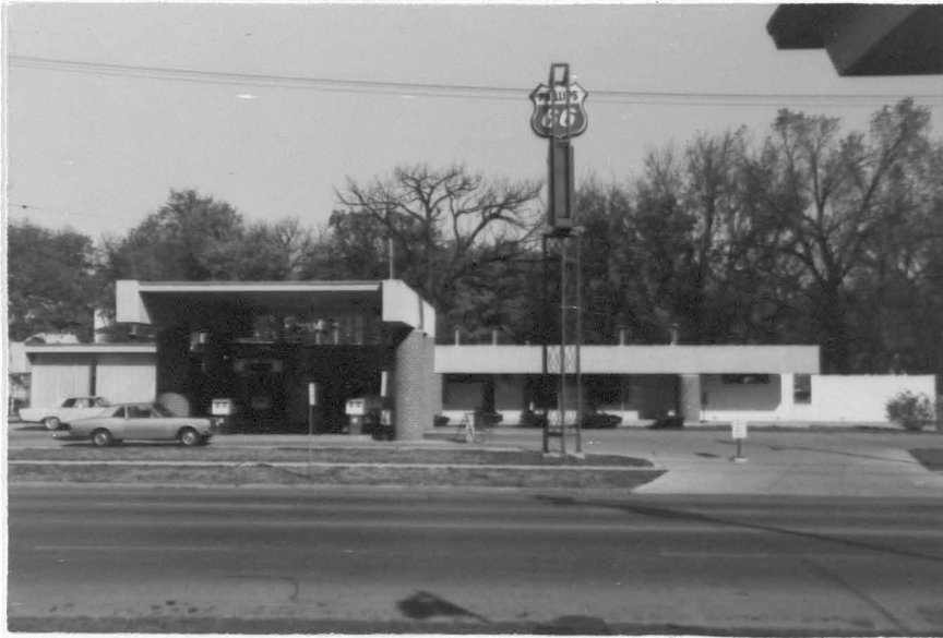
Figure 63. Ingersoll Car Wash looking north
