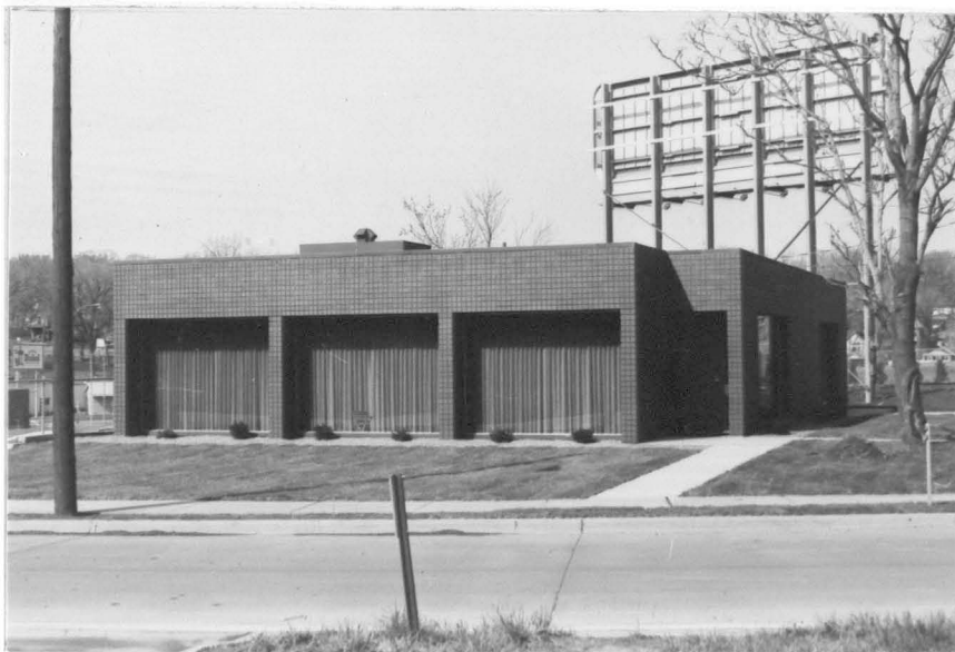
Figure 50. Des Moines Lighting looking southwest
