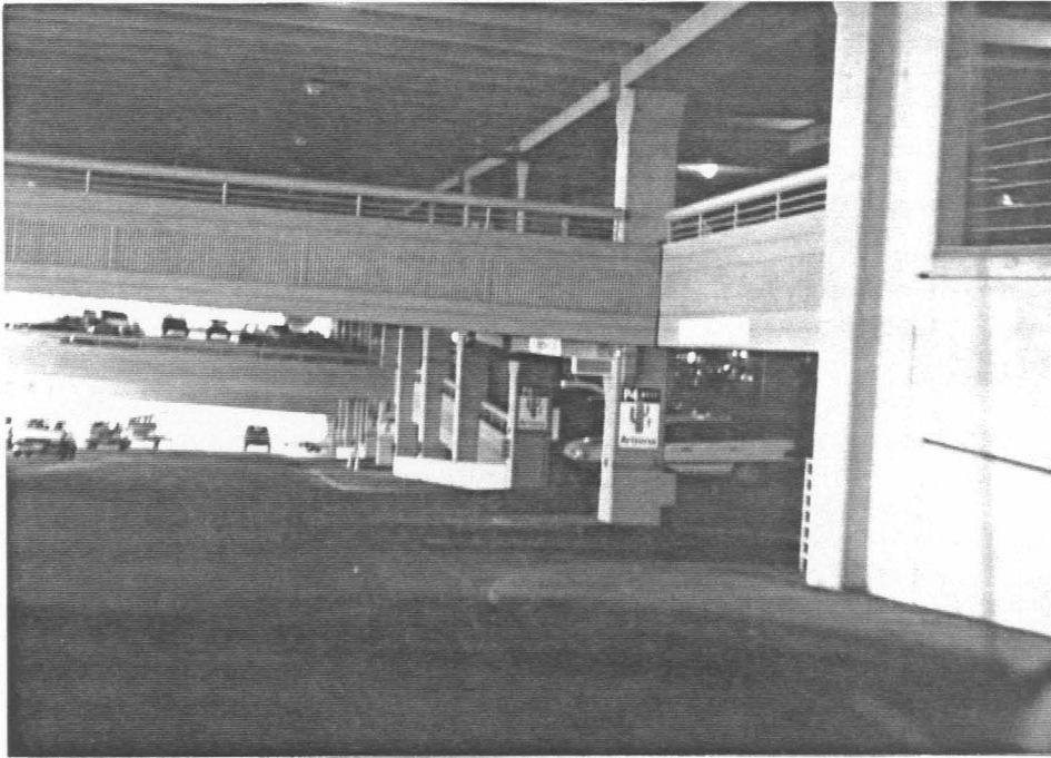
Figure 5. Parking lot ramp viewing towards exit.
